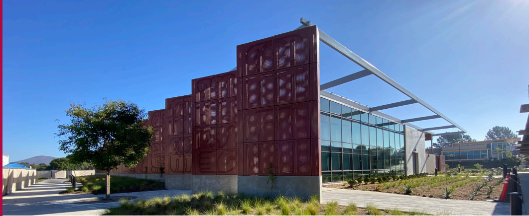
Glyphs outside IT Data Center Building.
