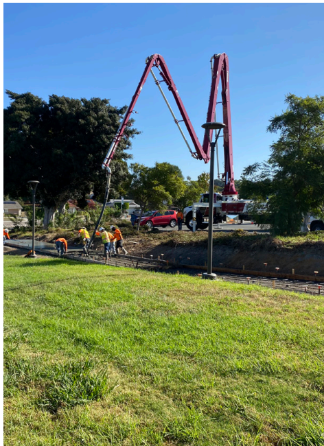
Upgrades to sidewalks and sewers.
